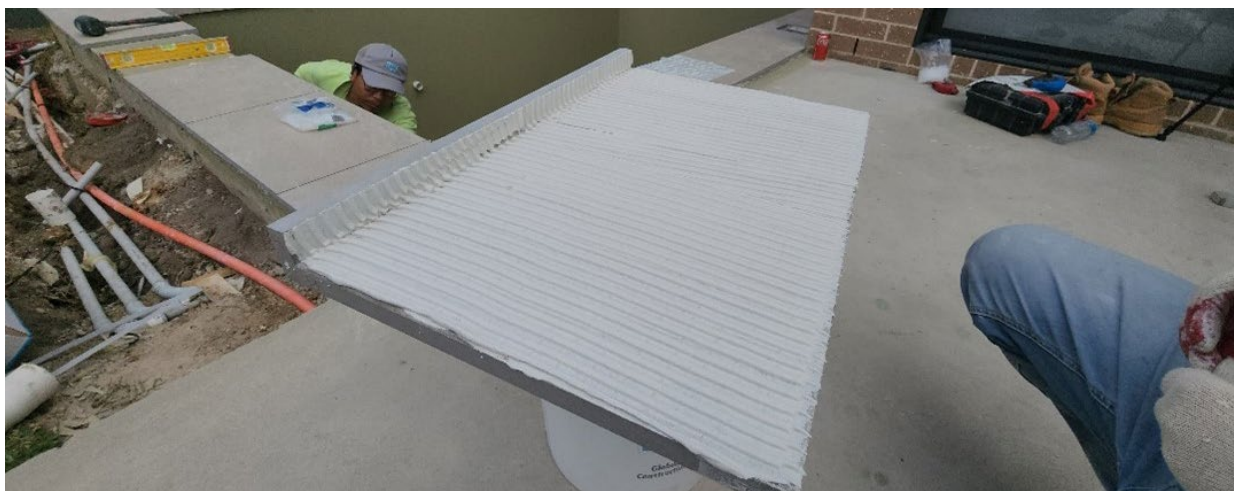
Image 4 - Back buttering 100% of the tile prior to installing onto substrate.
